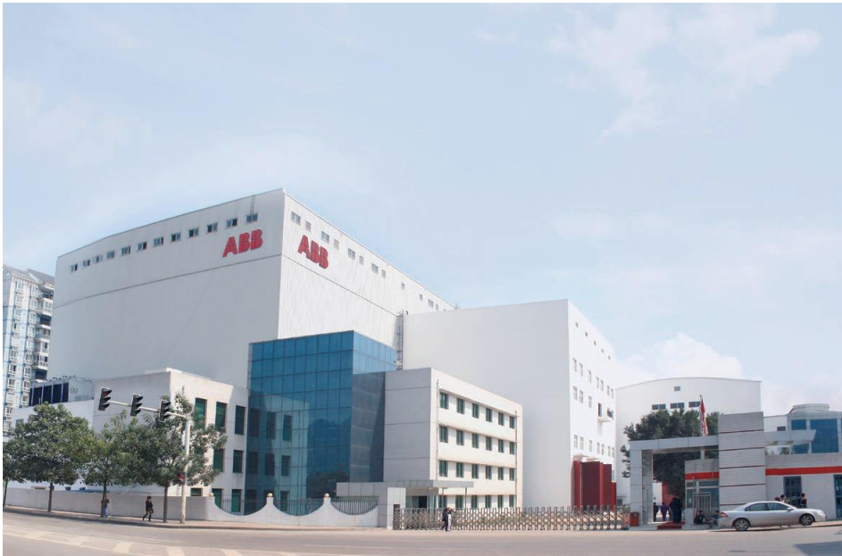
ABB China Engineering and Service Center
